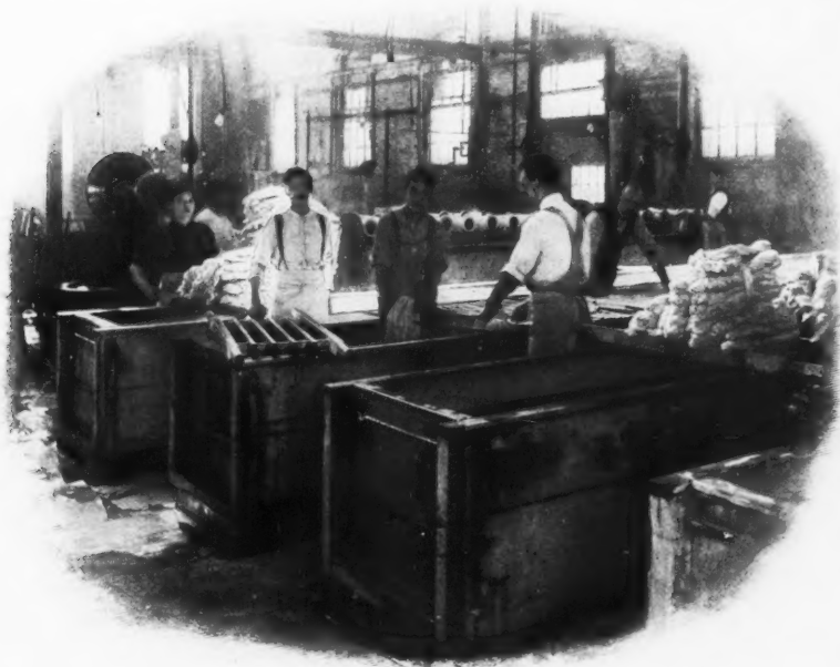
STRIPPING OR BOILING-OFF PROCESS, TO REMOVE THE ADHERING GUM.
